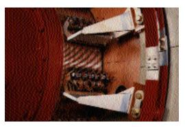
Massive reaction-type brush holders provide optimum commutation in DC applications.
